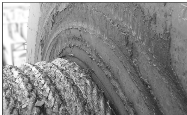
Fig.: Wear on a drum flange
